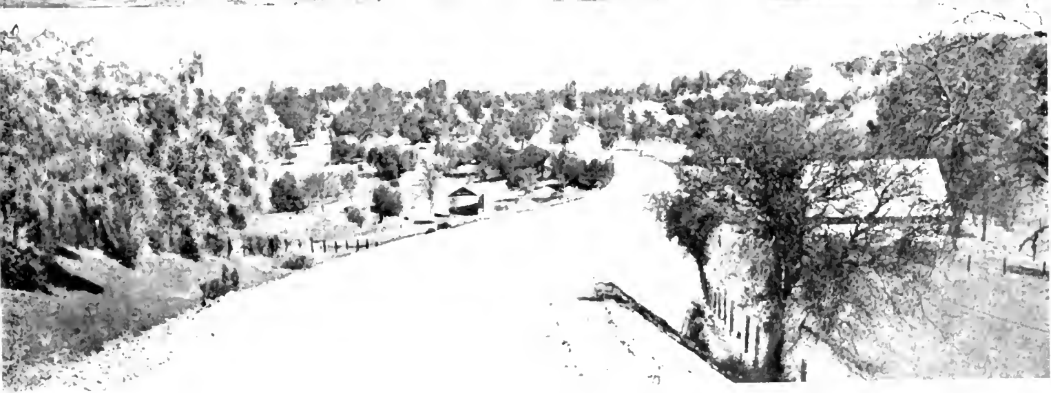
At top—lumber trucks hauling heavy loads over steep grades and sharp turns on old road east of McKeimpe Hill before realignment. Center—big load of logs tops summit of McFadden Hill on new, wide highway. Bottom—view east of Flume House Hill on State Highway 5 where 10 per cent adverse grade was regraded to 7 per cent.
